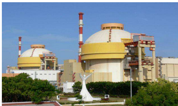
Fig. 2: Side View of Light water Reactor of KNPP in Kudankulam.
