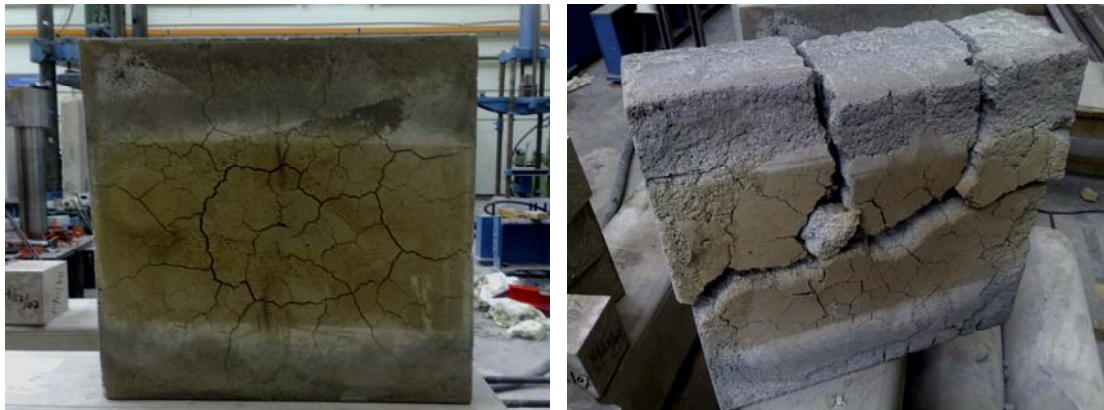
Fig. 11: Condition of prototype foamcrete panels after long hour's exposure at elevated temperatures on top of an electric kiln
