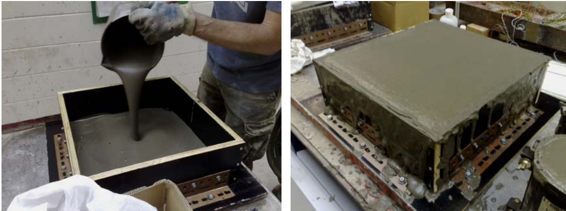
Fig. 10: Preparation of 650 \text{ kg/m}^3 density foamcrete prototype panel with dimensions of 430 mm x 415 mm in plan and 150 mm in thickness for small scale fore test.
